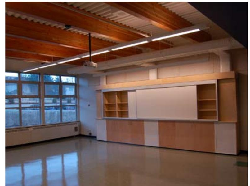
DISPLACEMENT VENTILATION: The wall cabinet, with sliding white boards, is designed to bring air ducts down to floor level. All classrooms also have audio enhancement systems.
